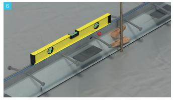
Ensure the adjustable bottom section of the divider plate is touching the slipo membrane on the sub-base. The ArmourJoints are now prepared and concrete can be cast against them. Using a small spirit level check the top edges of the joint are horizontal. Make adjustments to the joint via the wooden wedges to the the joint plumb.
