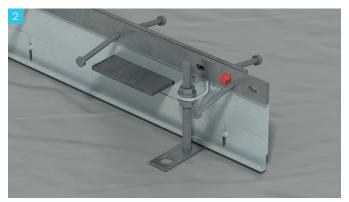
Fit the leave-in-place feet to the joint by removing the uppermost flanged nut from the foot, inserting the threaded bar of the foot through the lug which is welded to the ArmourJoint divider plate and re-fitting the flanged nut. Attempt to position the foot to the correct height approximately to reduce the amount of adjustment later.
