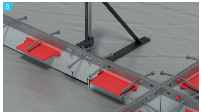
6 Continue to fit the ArmourJoints. Ensure the lapped joints are butted end to end tightly. Fit the plastic bolt and wing nut at the lapped joint.
