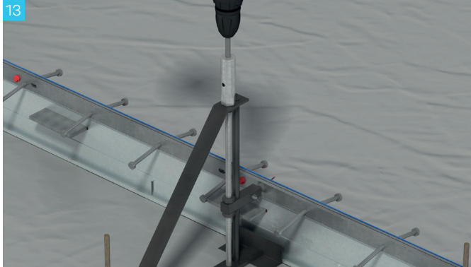
13 Final visual inspection, adjust the position and height of the joint if required.
