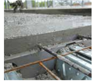
STEELDECKJOINT® FORMWORK
