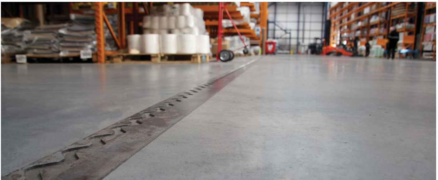
Completed Isedio Shieldjoint at Headlam.
